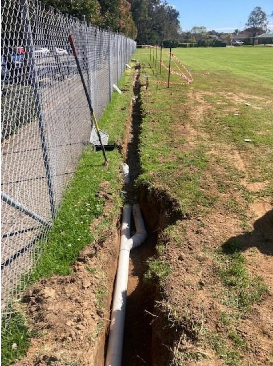
Figure 8: Drainage excavation in the study area
